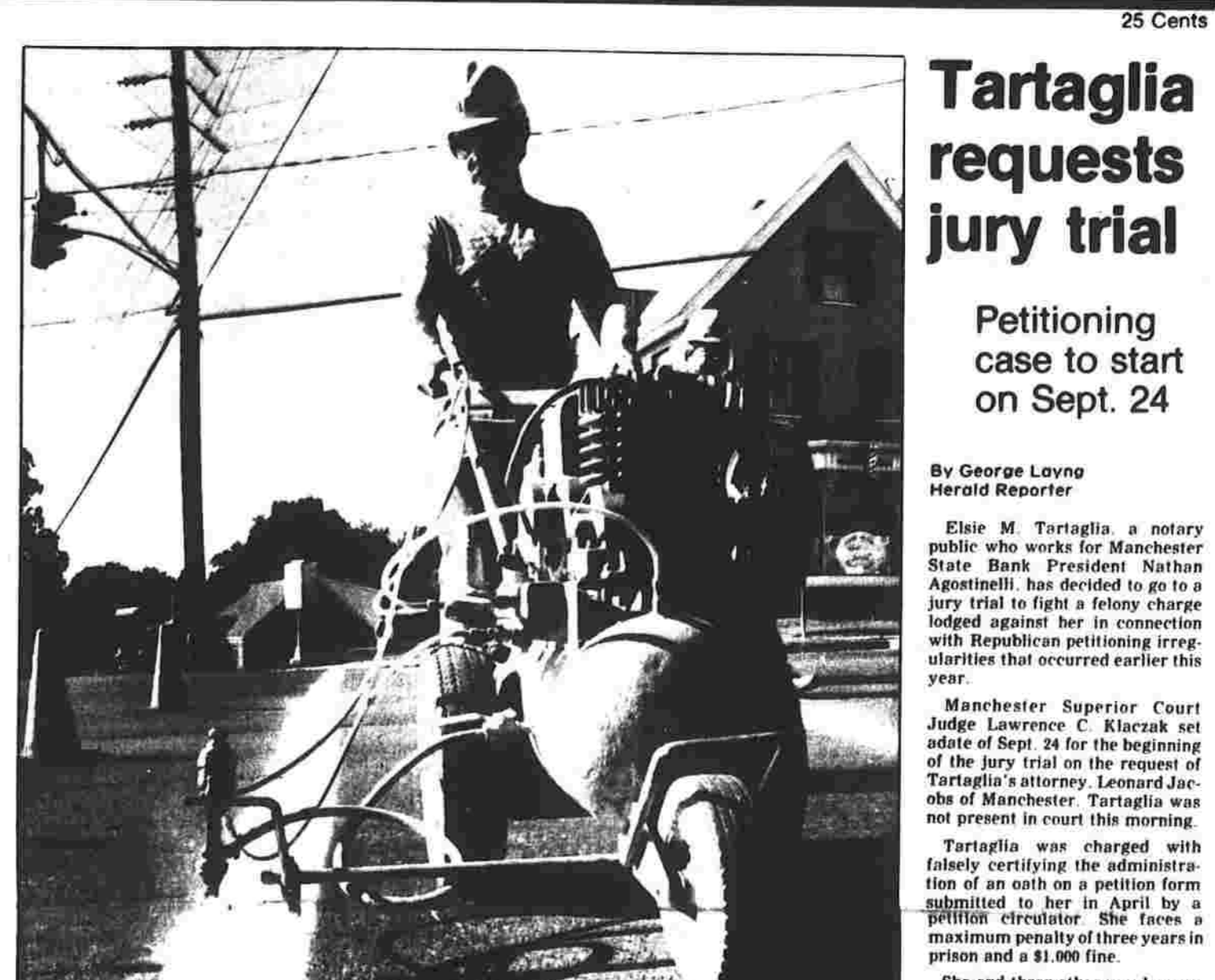
Laying lines... Douglas Bouvin sits on a line-painting machine as he sprays a white line on the road at the corner of Center and Stone streets Tuesday morning.
